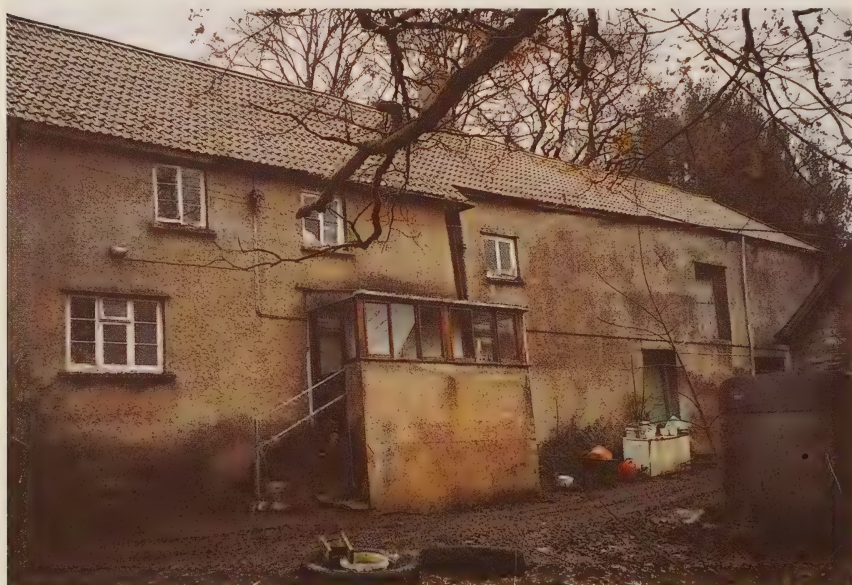
Brockhole, one of the remotest farms in Morebath: under the modern porch and pebbledash the layout of a medieval Devon longhouse is visible. People and animals shared a single roof on either side of a central entrance.
